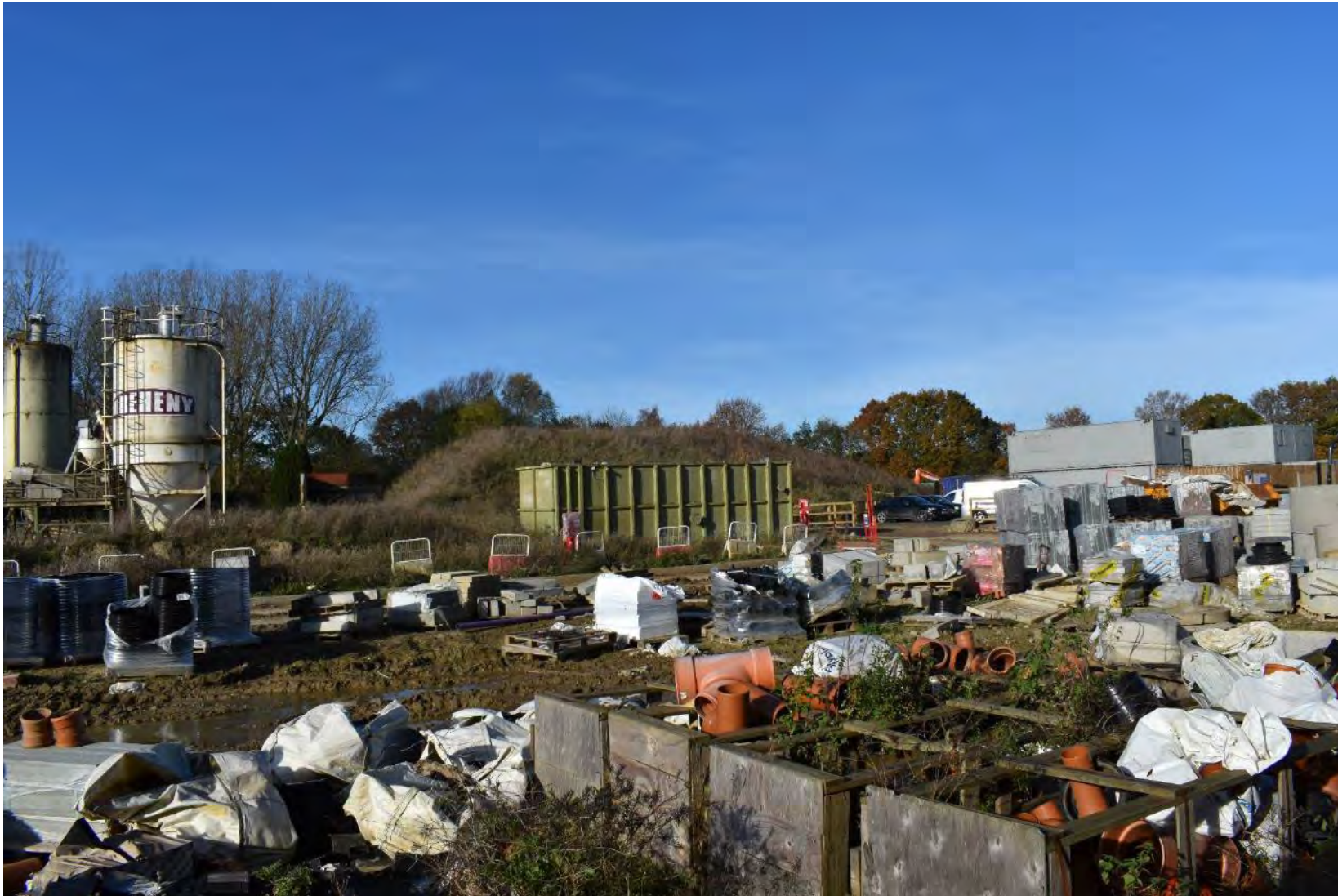
Plate 23: View across the northern part of the main section of the Application Site (facing W)
