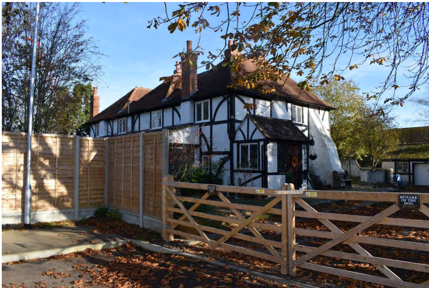
Plate 26: Conningbrook Manor (facing NE)
